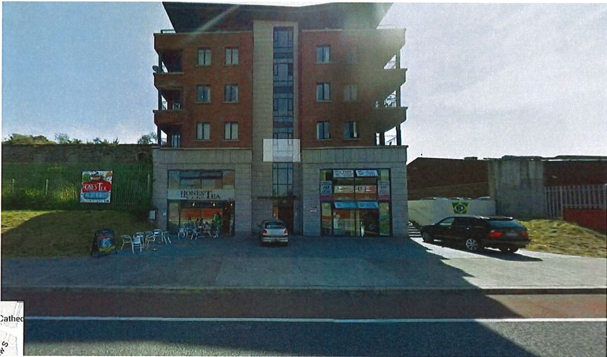
Fig 1: Subject land prior to improvement works at St Luke's Church and removal of redundant drainage chamber.
